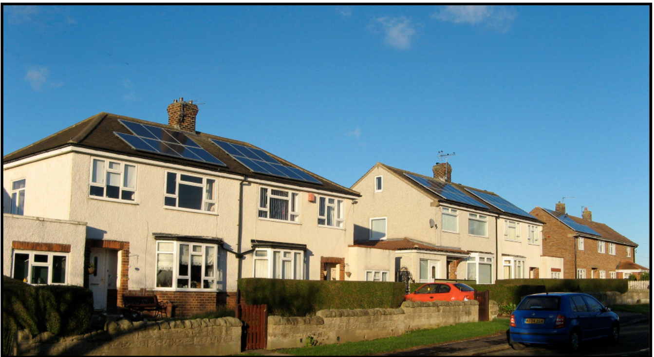
Five solar PV systems along Norton Road
