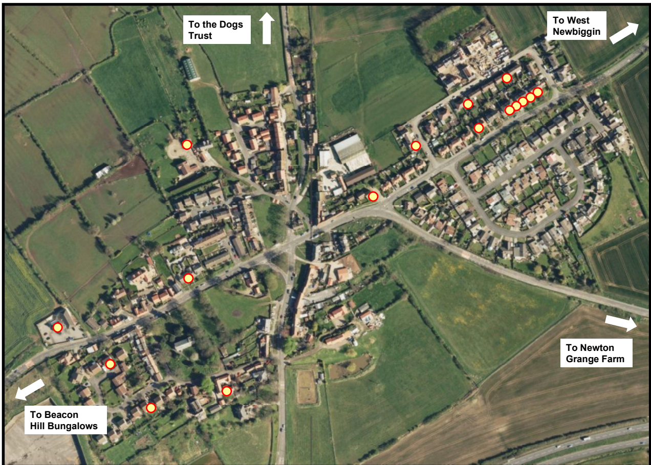
The locations of the 16 solar PV systems in Sadberge Village
